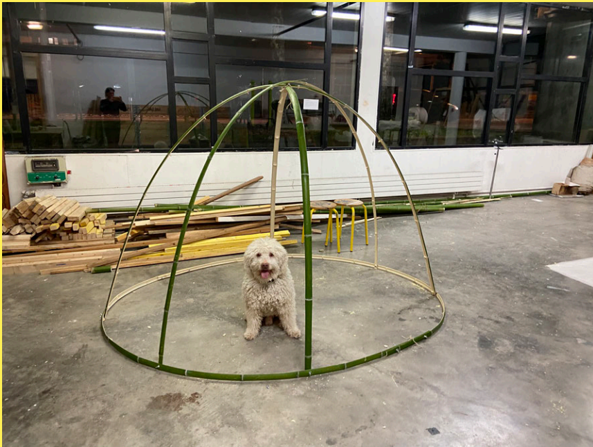
FIRST ATTEMPT TO BUILD A "KENNEL" WHICH FINALLY EVOLVED. TODAY, IT IS A GENOTAPH, THE HUSK
